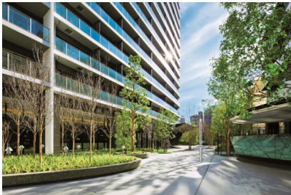
Energy-efficient glass is used in the windows to reduce the amount of sunlight and heat that enters, in this way alleviating the burden on the air-conditioning systems.
